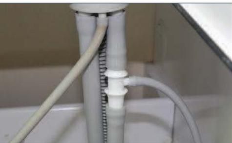
*\*An alternative option is to cut a small section (1/2") of the 6' suction hose where the HVE adaptor is connected if you have trouble removing it manually.*
